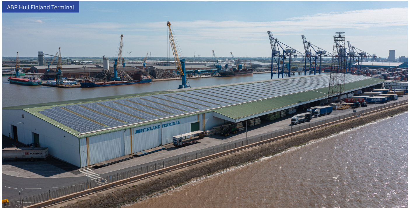
ABP Hull Steel Terminal
