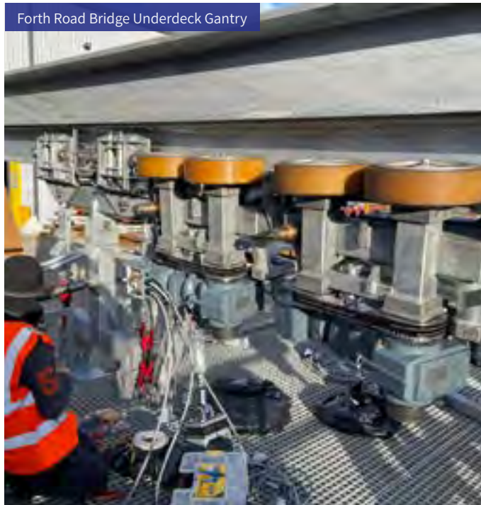
Forth Road Bridge Underdeck Gantry
