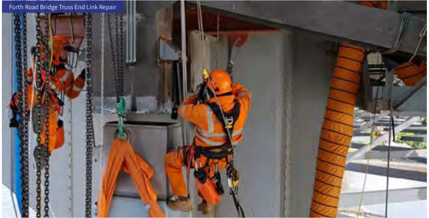
Erskine Bridge Steelwork Repairs
