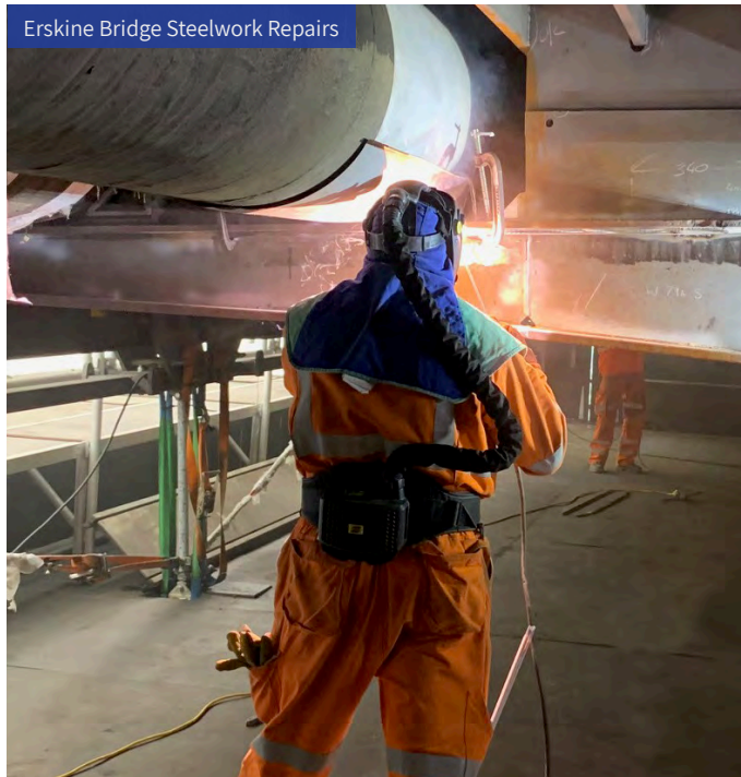
Erskine Bridge Steelwork Repairs
